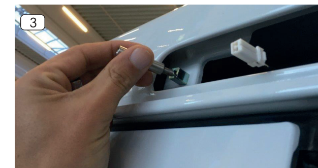
3. Screw in and tighten the stainless steel mounting bolts by hand (5Nm). Use a dab of Loctite, if possible.
